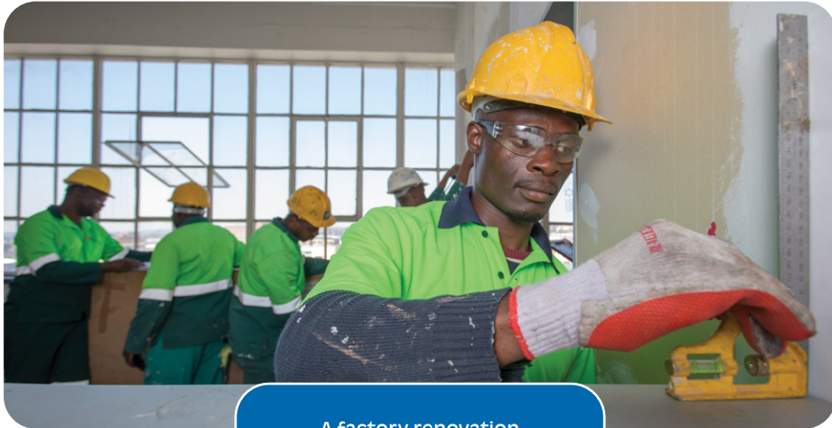
A factory renovation
